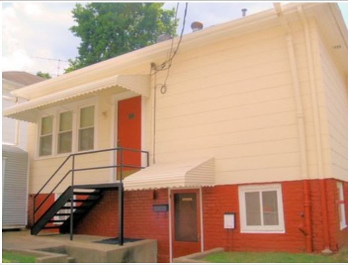
Close Up Of Private Rear Entry Door To Su...
