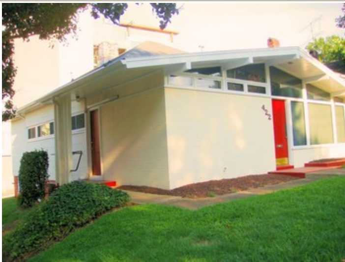
Front Left Corner Of Building On Saint Mar...
