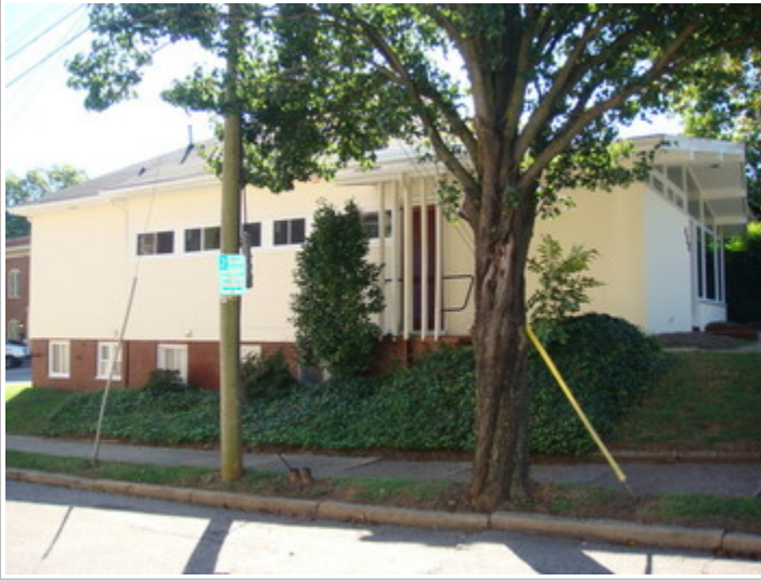
Entrv Door To Suite 6 - Front Side of Buil
