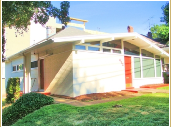
Front Left Side Of The Building
