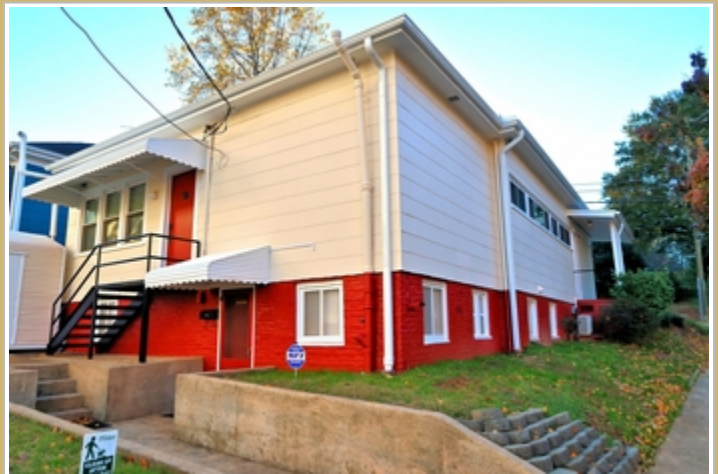
Another View Of Rear Of Building
