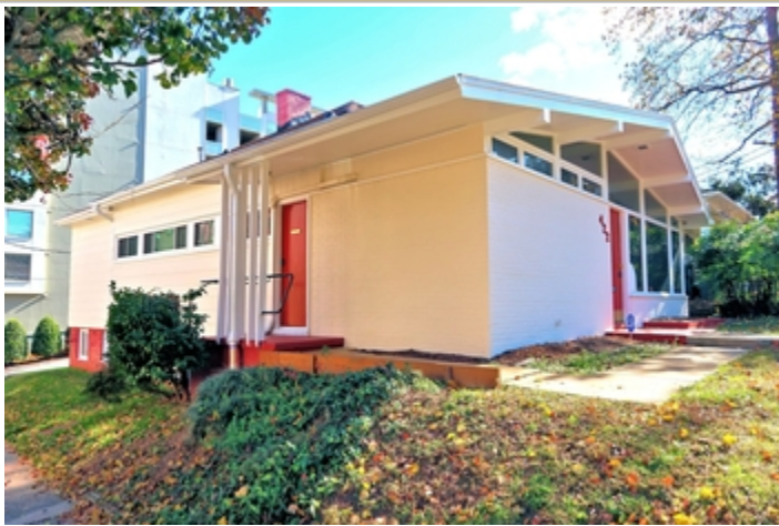
Front Left Corner Of The Building
