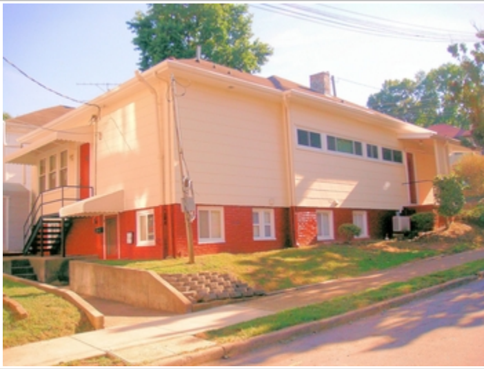
View Of Left Corner And Rear Of building
