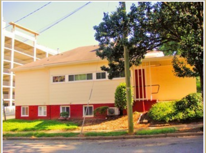
Side Of The Building From Tucker Street
