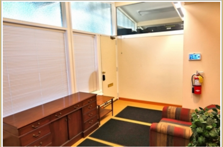
View Of Front Entry Door To Lobby
