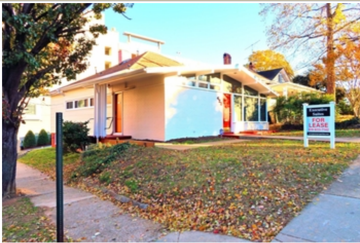
View Of Building From Saint Mary's Street
