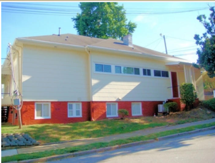
Another View Of Side Of The Building
