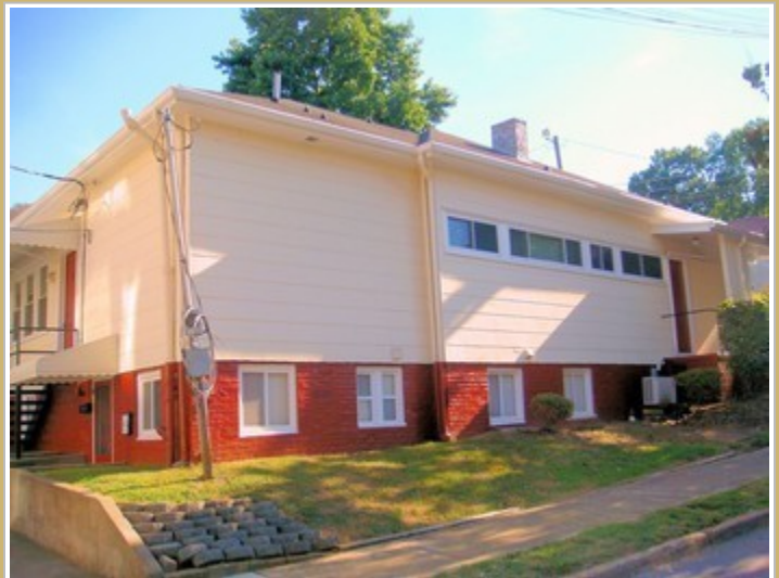
View Of Left Corner Of Building
