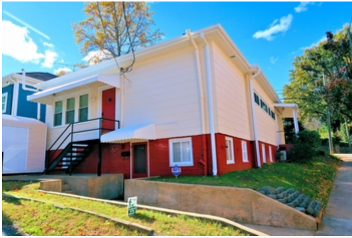
View Of Rear Of Building And Sidewalk
