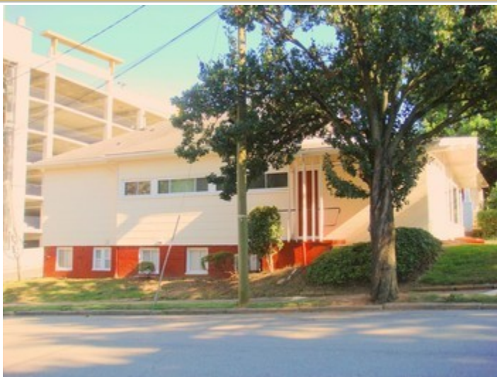
Side Of The Building
