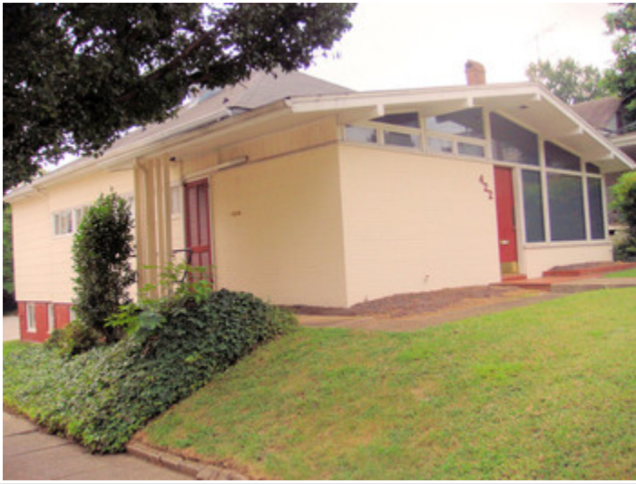
Front of Building
