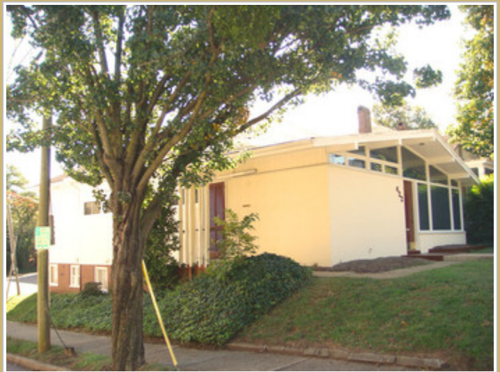
Front Corner of Building
