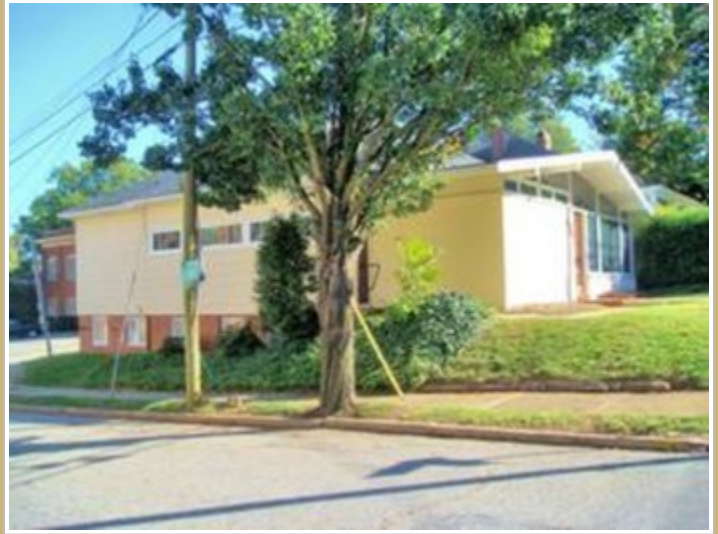
Front Corner Of Building
