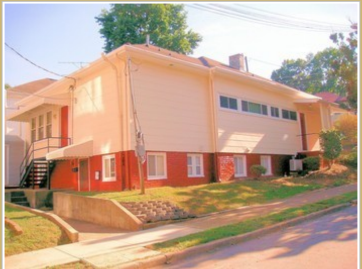
Rear Corner Of Building
