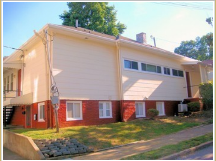
Side Corner Of Building
