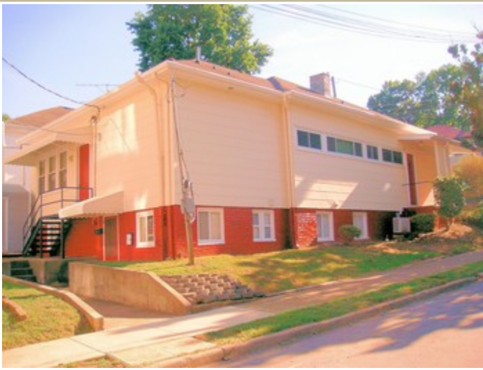
Rear Side Corner Of Building
