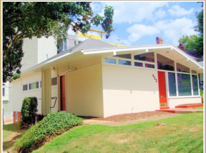
Left Front Corner View Of Building
