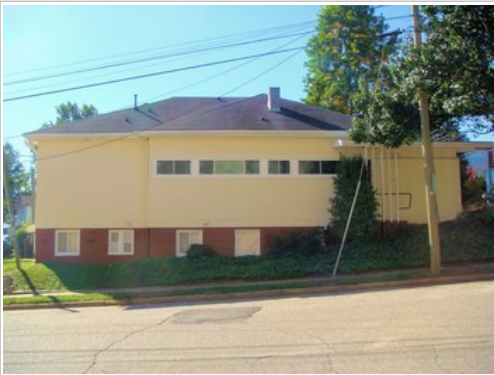
Left Side of Building
