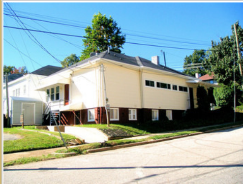
Rear Corner of Building
