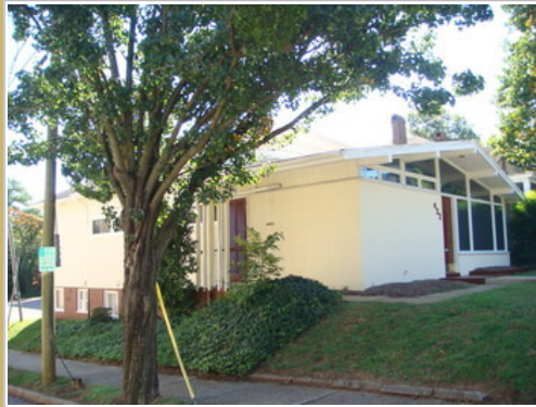
Front Corner of Building
