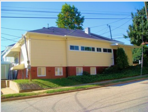
Side of Building with Vinyl Windows
