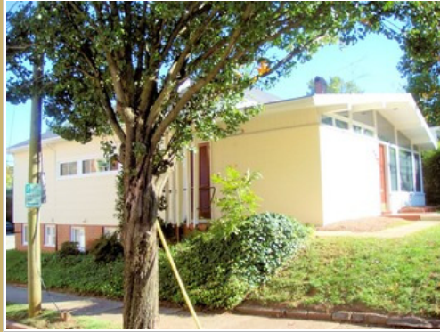
Left Side Building
