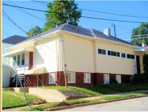
Rear Corner of Building
