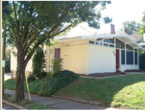
Front Corner of Building
