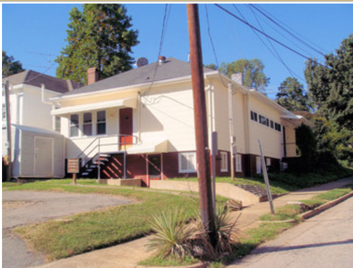
Back Of Building
