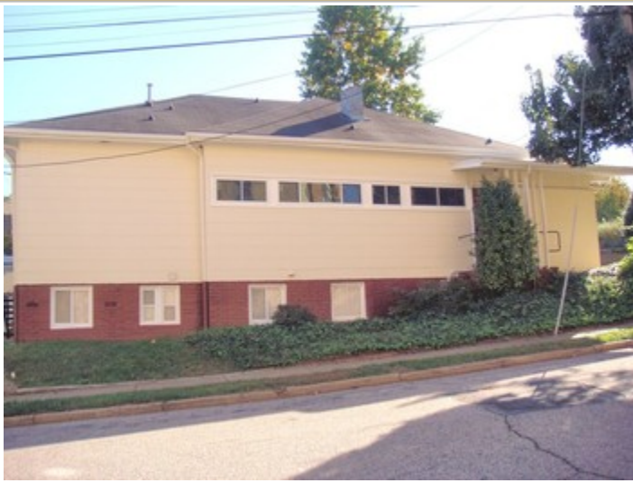
Side of Building
