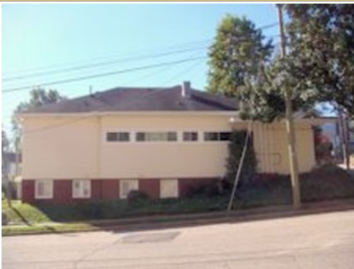
Side of Building facing Tucker Street
