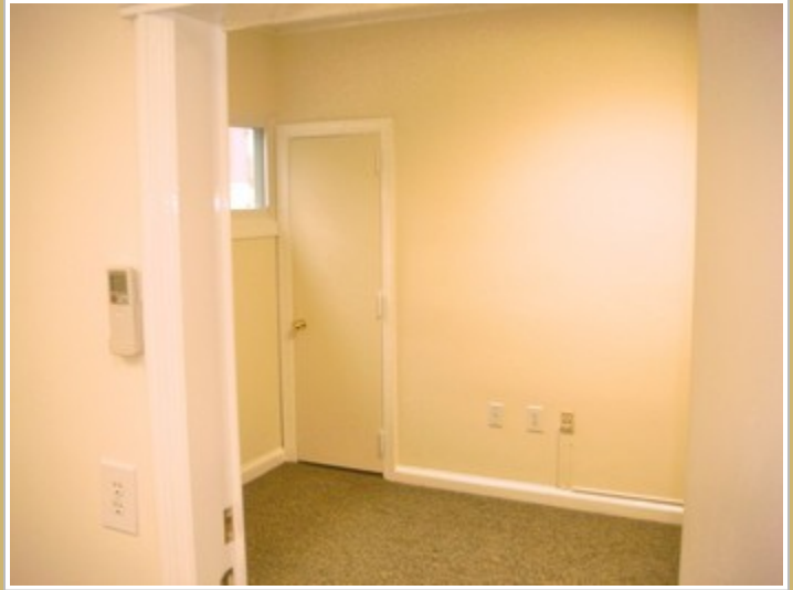
View of Office 1 from Office 2
