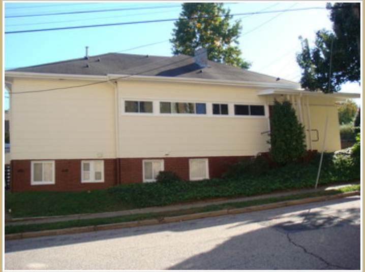
Side of Building facing Tucker Street
