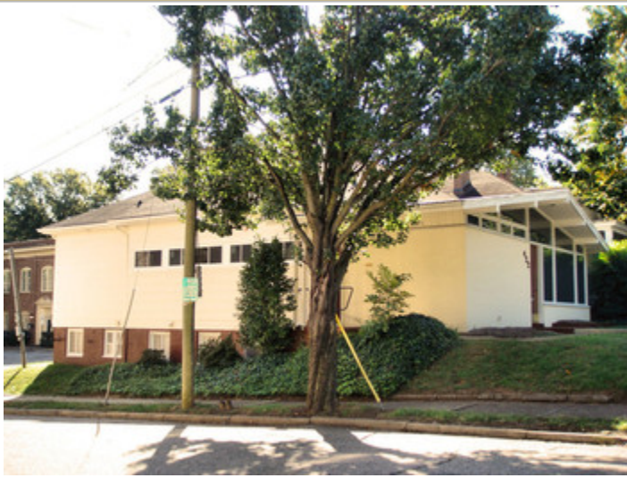
Front Corner of Building
