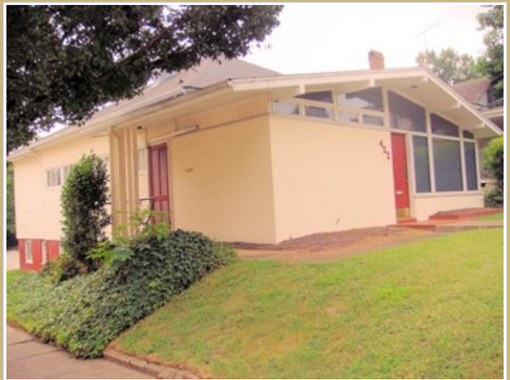
View of Entry Door to Suite 6
