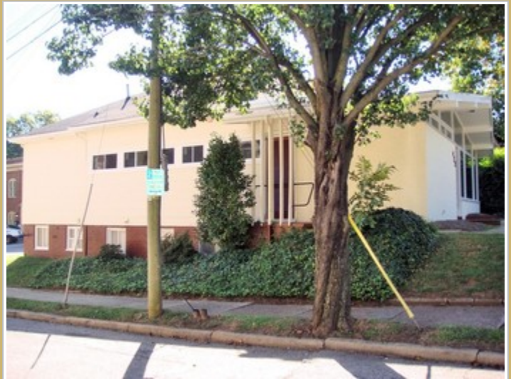
Side of Building - Entry Door to Suite 6
